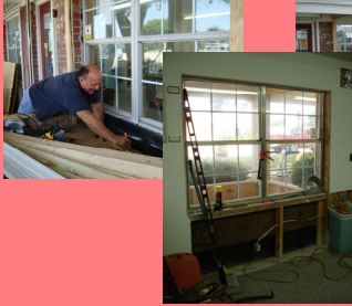
Craig Augustine building the shark tank.
